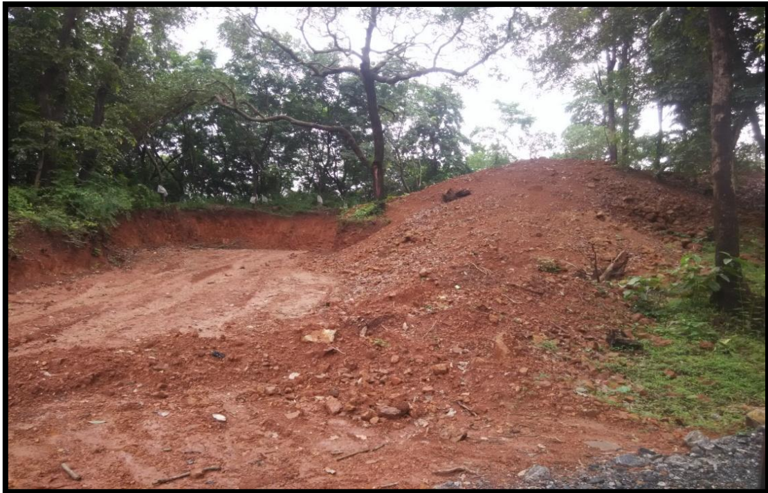
Top soil stacked in project site
