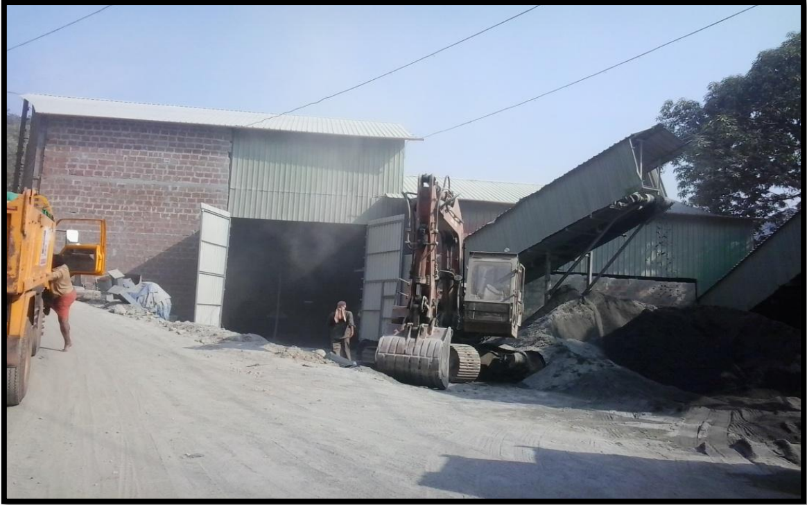
Crusher in the project land
